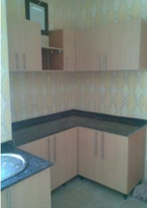
Figure 7: Composite materials used in the production of a kitchen medium density fibre [MDF] for the panels and other composite for the kitchen countertops
