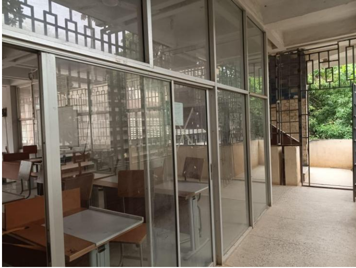
Figure 5 Aluminium usage for partitioning of space Ahmadu Bello University 2 nd Year Studio:
